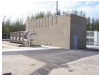
Upgrade of fuel storage and distribution
